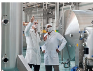
Pharmaceutical water treatment
